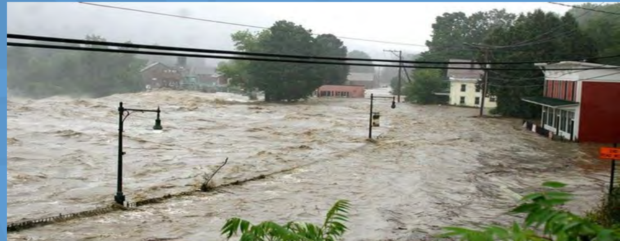
Flooding on Conway St., Buckland, MA Photo: J. Brown
