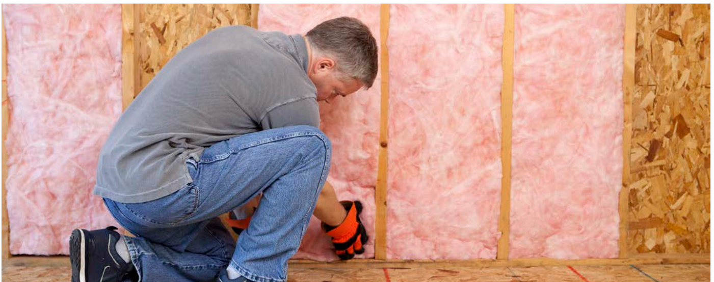
FIGURE 24: Ensure contractors know program retrofit standards.
