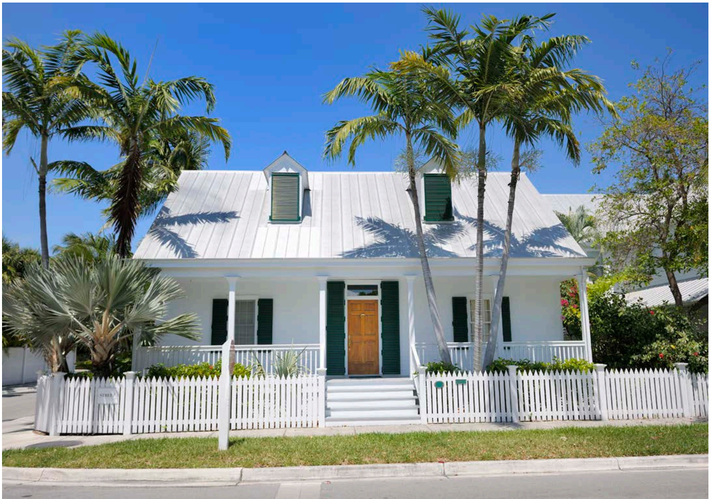
FIGURE 2: Programs can be tailored to address the community’s risks, vulnerabilities and natural hazards.
